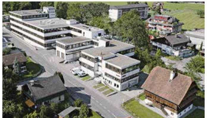
Leister Technologies AG, factory, Kaegiswil, Switzerland
