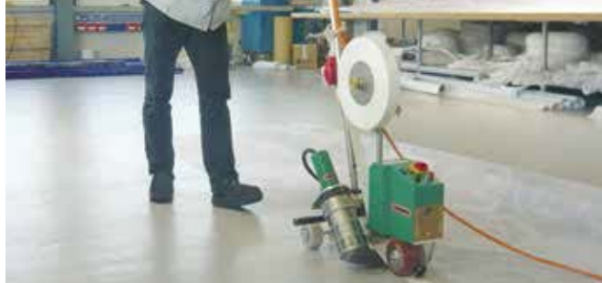
Welding tape at maximum speed.
