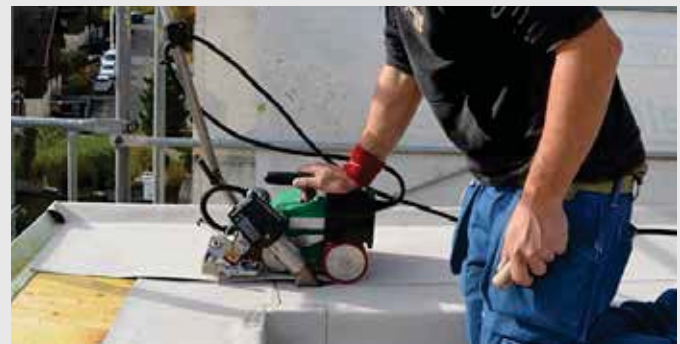
Clean overlap welding of base welds.
