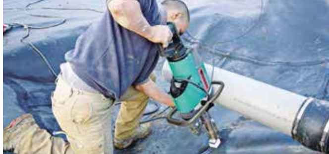
WELDPLAST S6 undertaking assembly applications on a landfill site.
