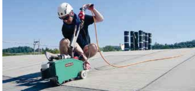
Flameless welding of modified bitumen with the BITUMAT.
