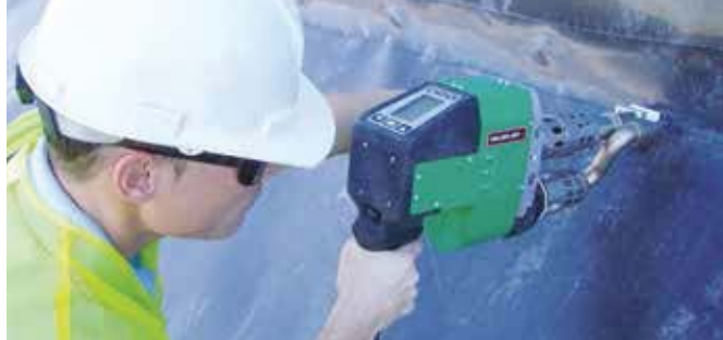
The powerful WELDPLAST S4 at work.
