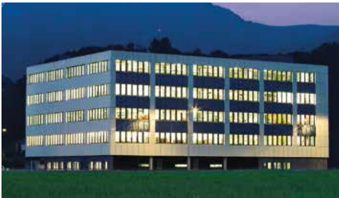
Leister Technologies AG, factory, Sarnen, Switzerland
