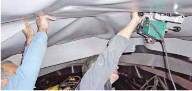
Comet operating in the tunnel ...
